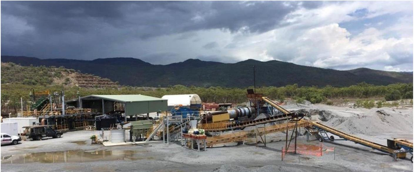
View of the commissioning of the Retreatment Plant (raw material intake at front right; screening, crushing and jigging at center front; gravity circuit under shed).
